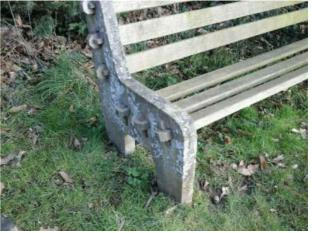
The bench is not securely fixed to the surface **Action:** and there is some possibility of the item tipping or rolling over Finding:
