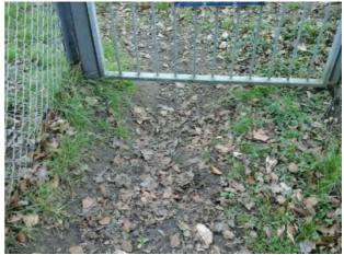
Finding: The area under the gate has eroded leaving uneven areas, or the concrete foundations exposed, resulting in trip hazards at the entrance/exit to the playground
