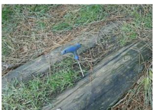
Finding: There is some evidence of rot in the timber balance beams
