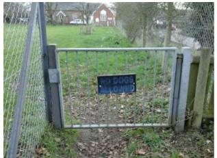
The gate is not a contrasting colour to the fencing making it difficult for users with impaired sight to distinguish it from the fence Finding:
