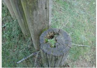
Finding: A number of The palisade logs have rotted Action: Replace all affected timbers
