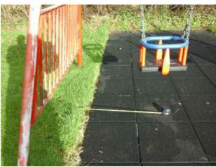
The surfacing width under each seat is less than 1.75 metres and fails the requirements of BS EN 1176 Part 2 Finding:
