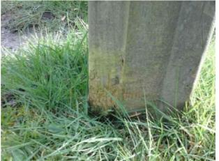
Finding: There is some strimmer damage apparent on **Action**: the posts, this can penetrate the preservative applied to the timber and accelerate the rotting process
