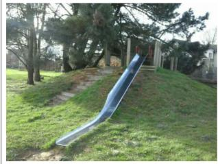
The slide start section incline is not in the direction of travel; it should slope towards the direction of the sliding surface Finding:
