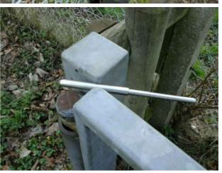
**Finding:** The opening between the gate and the post is **Action:** less than 12mm and could trap users fingers
