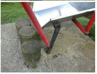
Parts of the steel on this item have corroded excessively and the metal has perforated in Finding:
