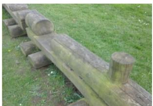
Finding: The timber has a number of air cracks apparent, the splits will have penetrated the preservative applied to the timber and allow water ingress to the unprotected areas
