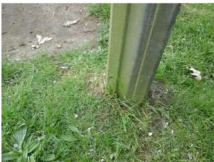
There is some strimmer damage apparent on the posts, this can penetrate the preservative applied to the timber and accelerate the rotting process Finding:
