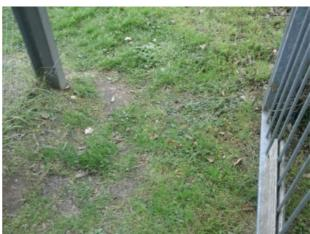
The area under the gate has eroded leaving uneven areas, or the concrete foundations exposed, resulting in trip hazards at the entrance/exit to the playground Finding:
