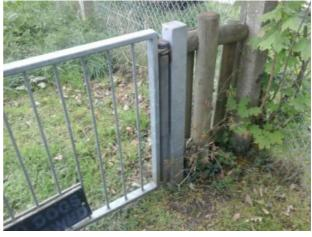
Finding: The gate is closing too quickly (less than 4 seconds)
