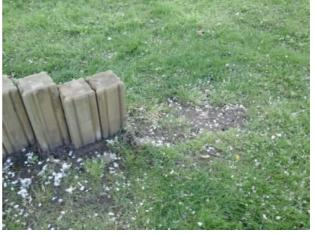
Finding: The surface has eroded and the foundations Action: Reinstate surrounding surfaces to cover the foundations
