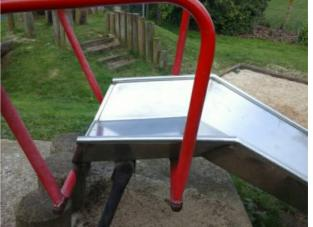
Finding: The slide start section incline is not in the direction of travel; it should slope towards the direction of the sliding surface
