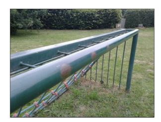
The paintwork on this item has been damaged or worn exposing the metal Finding:
