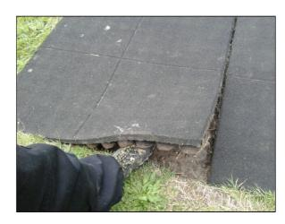
Finding: The tiles can easily be lifted or are lifting along the edges of the area
