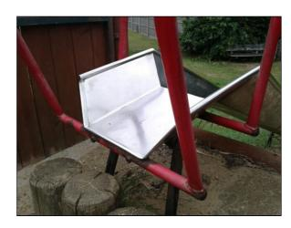
The slide start section incline is not in the direction of travel; it should slope towards Finding:
