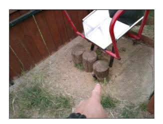
**Finding:** There are areas or parts of the timber on the structure that have rotted
