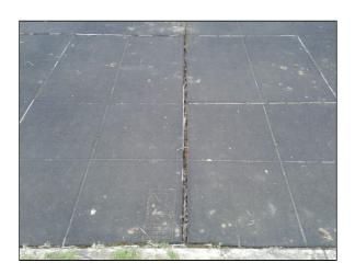
There are significant gaps (over 30mm) between the surface and the edging or between the joints in the surface; these are large enough for a small foot to enter Finding:
